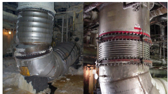
Replacement Metallic Expansion Joint Fabricated and Installed Within Two Days
