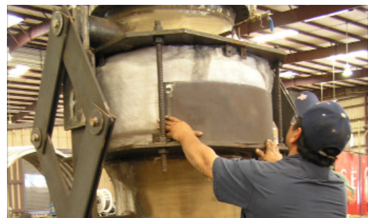
Installation of a Protective Cover on an Expansion Joint
